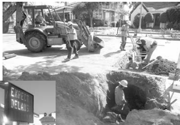
John Wood/Daily Press Above: A construction crew tends to a sewage line under Fourth Street on Tuesday afternoon. Parts of Fourth Street have been closed since Feb. 9 so the city can repave and complete work on water mains, curbs, sidewalks, the median, landscaping, crosswalks and signs. Below: Residents will have to wait longer through the summer, as work is expected to be completed by Sept. 30.
